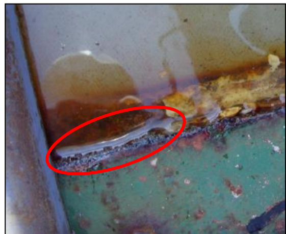
Figure 17: Silicone applied to the sealing faces
