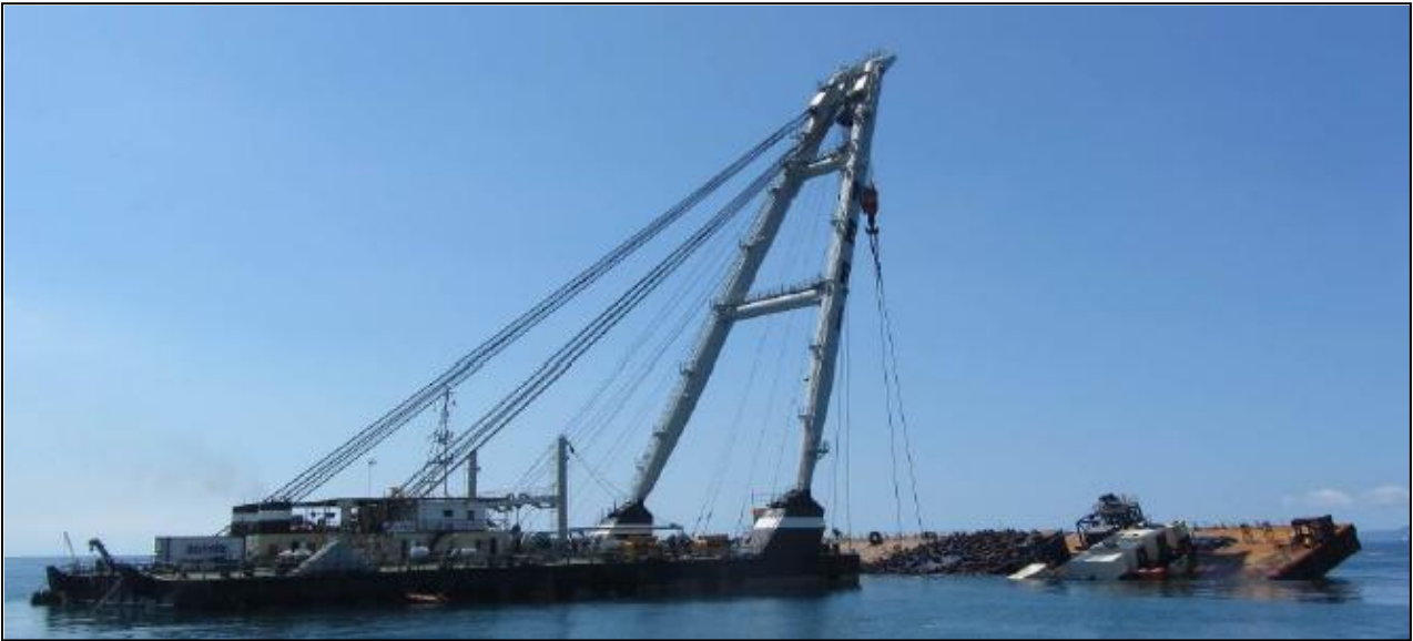
Figure 7: AMT Explorer connected to the parbuckling slings
