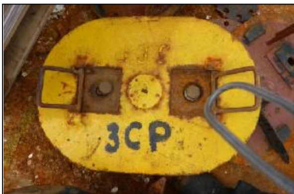
Figure 9: A manhole cover showing on bolt on each strong-back
